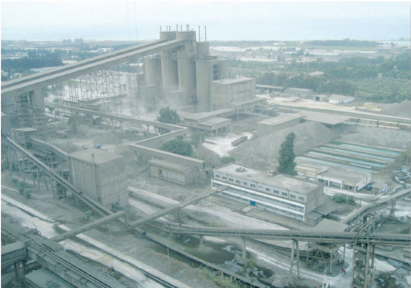
Figure 5: Cement plant without dust filters (installed by now), Syria, 2010 (MVW)
