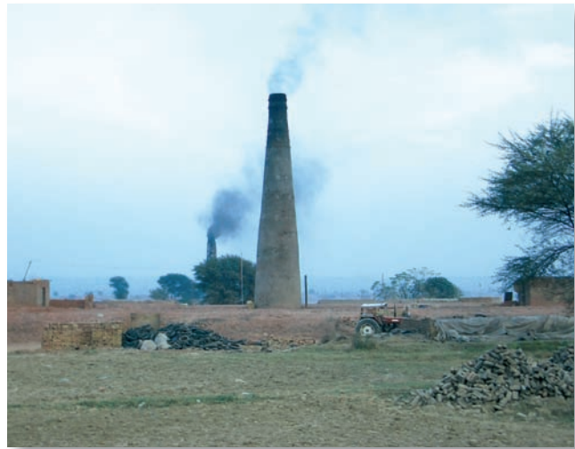
Figure 8: Old brick plants; burning waste as fuel without any emission control, Pakistan, 2007 (MVW)
