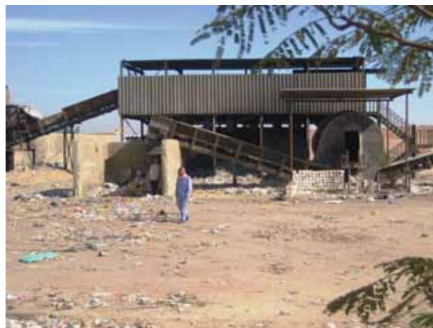
Figure 3. Waste processing plant in Egypt.
